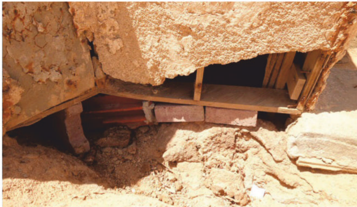
02 New bricks now underpin the Homestead's wooden substructure to protect it from water saturation.
